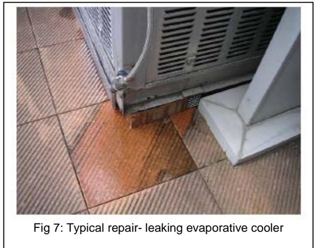
Fig 7: Typical repair- leaking evaporative cooler
