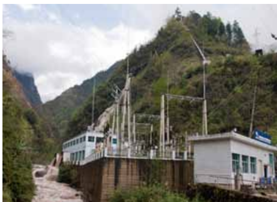
Outside view of Lishadi hydro plant
