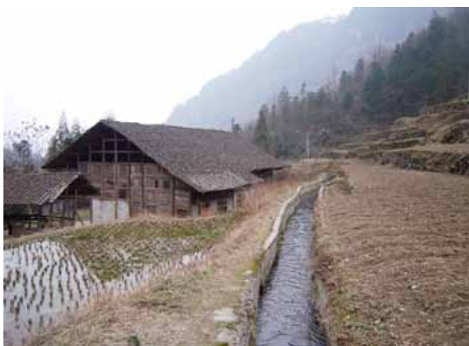
This canal is used to divert run-off water for the irrigation of agriculture terraces
